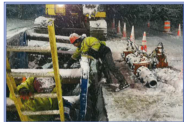
The night-time installation of a 3-way valve cluster during a snow event in Hyannis
